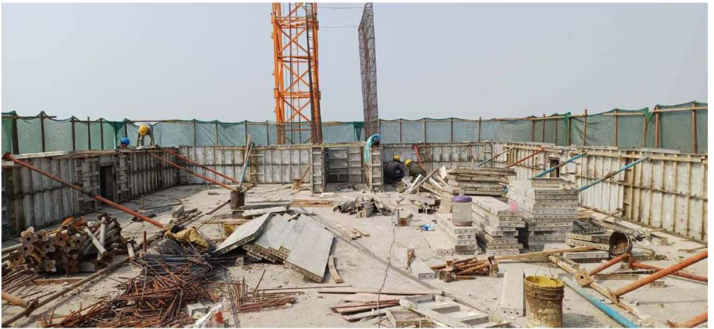
TOWER-2 ABOVE ROOF PARAPET WALL SHUTTERING WORK IN PROGRESS
